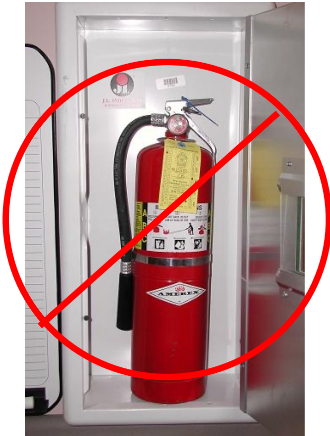
Red tank not MRI Compatible. Do not bring into the scanner room
