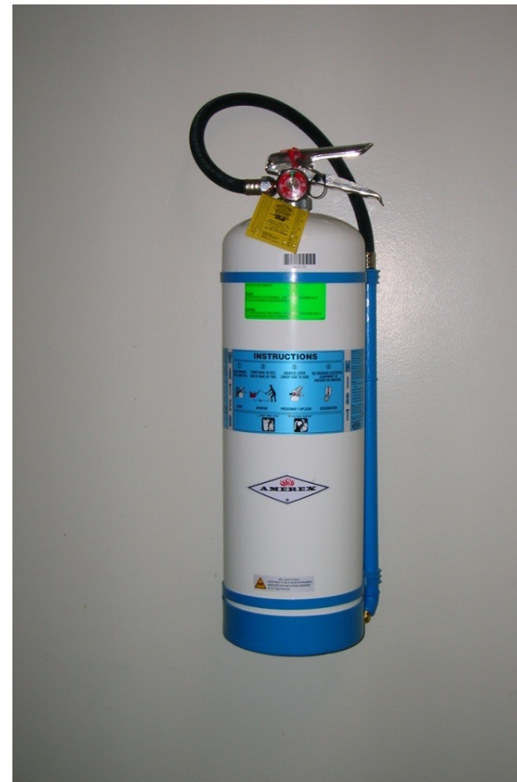
White or silver tanks are MRI Compatible. Can be brought into the scanner room
