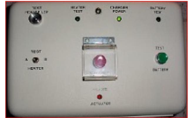
1.5T Scanner room Quench button
