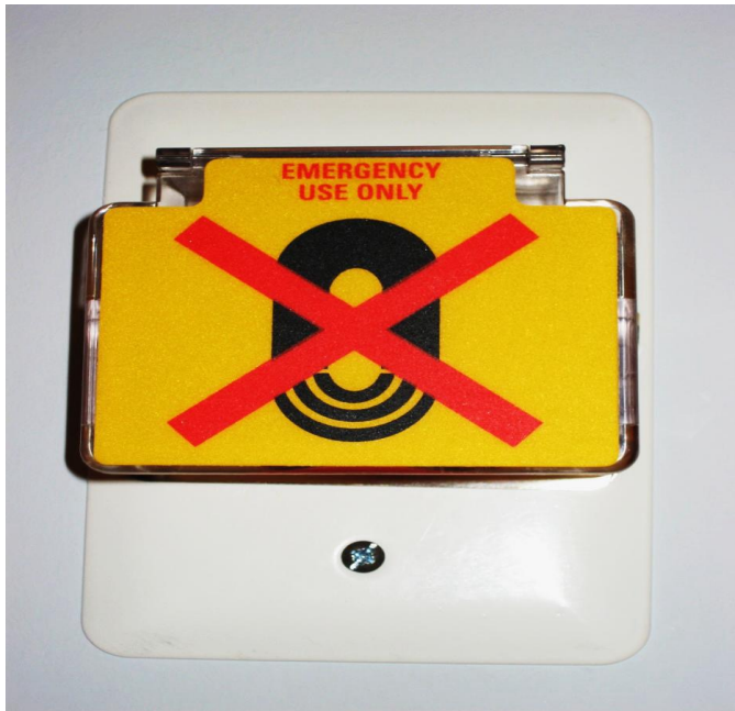
3T Scanner room Quench button
