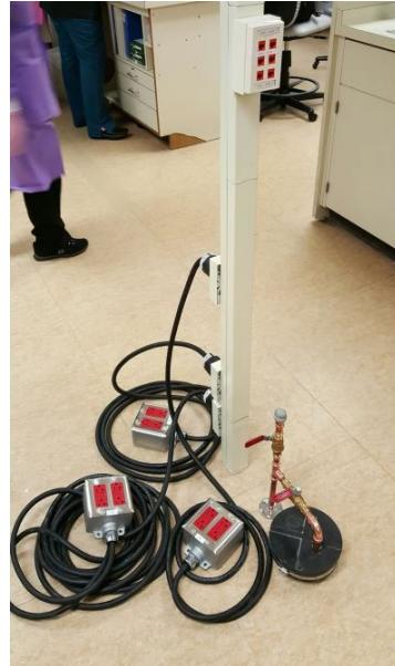
The customer should provide power to the XN-9100 system by way of dedicated circuits (117 V, 20A circuits, NEMA 5-20 type outlets). Typical sources of power are power poles, structural columns, floor mounted outlets, or an adjacent wall. The installation specialist will work with the customer to determine the best placement for the system and location of power.
