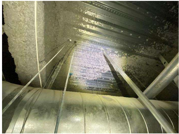
View of the sprayed-on fireproofing on the metal fluted deck and overhead beams
