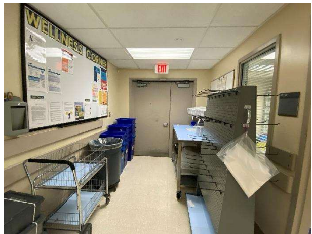
View of the floor tile and acoustical ceiling tiles throughout
